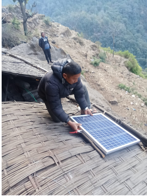
Figure 2: Engineer Bahadur Sing Limbu overseeing the installation of the 40 W solar system at the project site.
